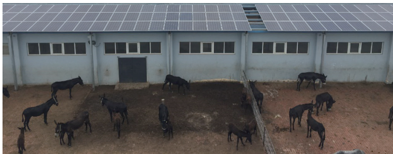
Photovoltaic donkey shed
